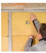
STEICO*flex 036* for interior insulation and for service voids
