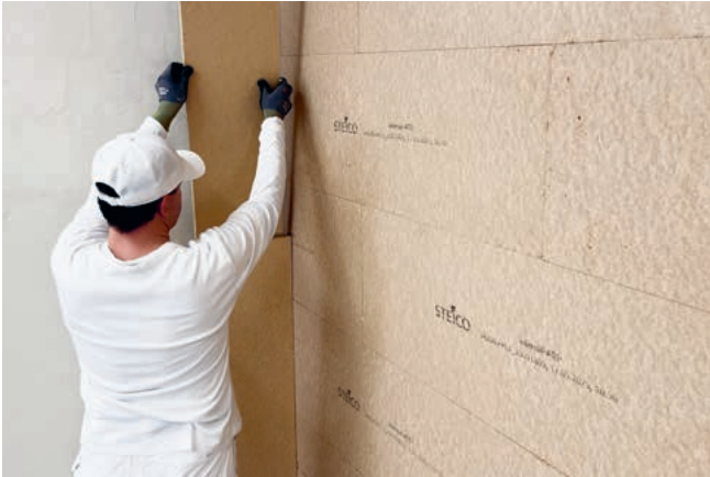
STEICO tri for side insulation
